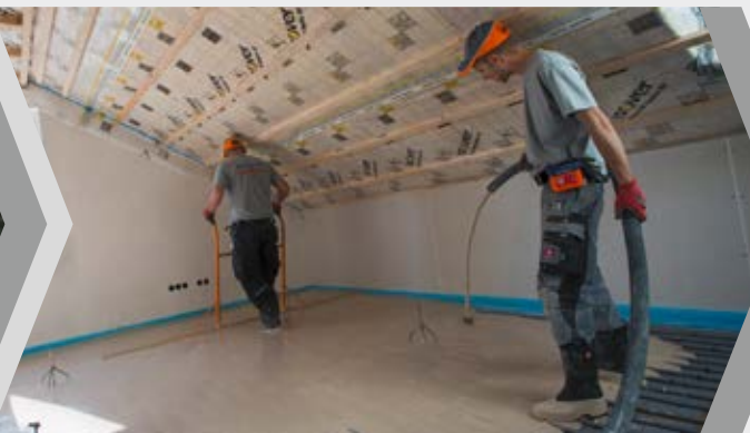
Placement of either self levelling floor screed (TransMix 3200) or semi-dry floor screed (TransMix 5500) – controlled by remote control
