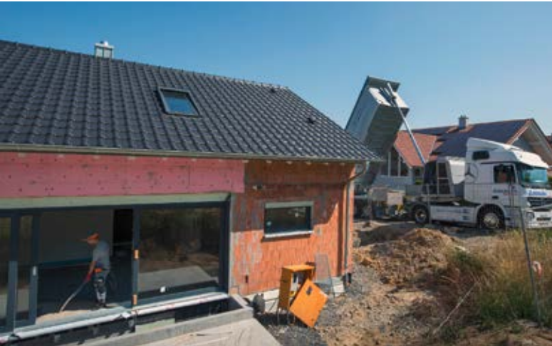
Placement of calcium sulphate based self levelling floor screed in a detached house using a TransMix
