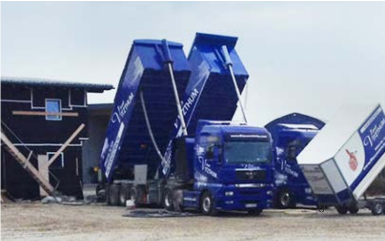
Site with polystyrene pour-in insulation
