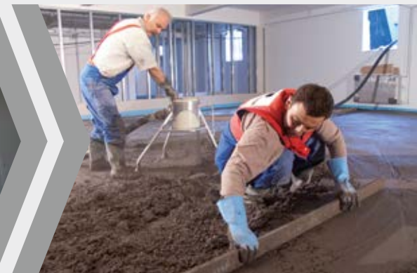
Placement of either self levelling floor screed (TransMix 3200) or semi-dry floor screed (TransMix 5500) – controlled by remote control
